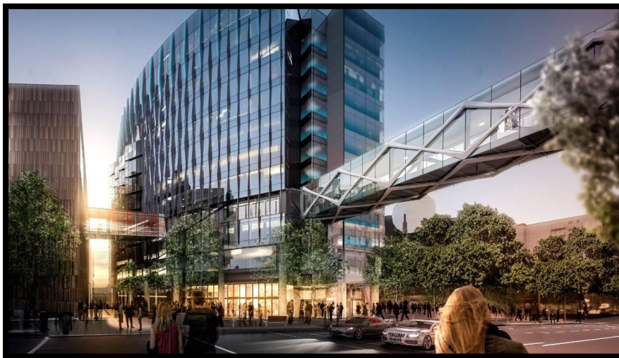
SkyCity's new Horizon Hotel in Auckland, under construction, is expected to open in 2020 and will have 303 rooms.
